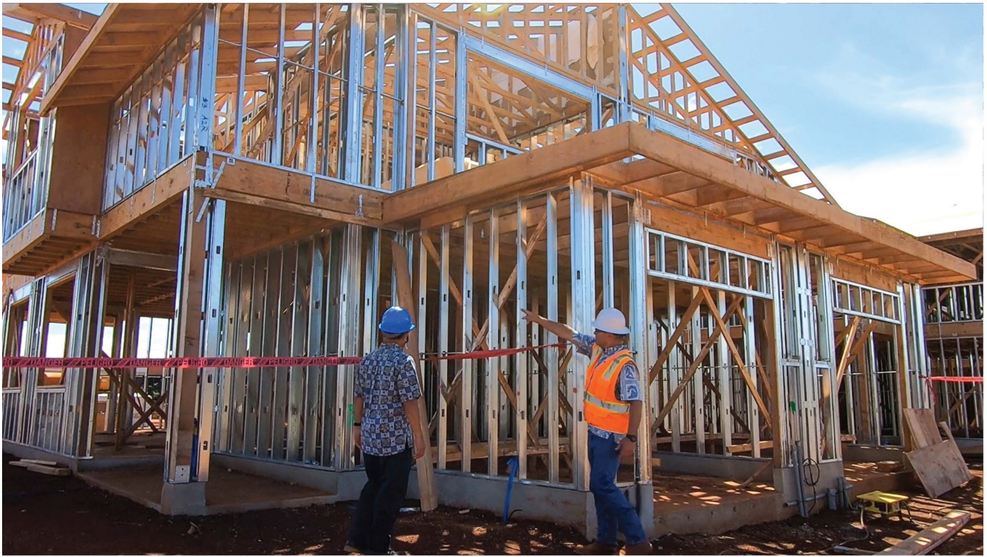
Castle & Cooke noted the hybrid system of engineered lumber and steel framing provides the benefits of strength, durability and support.
